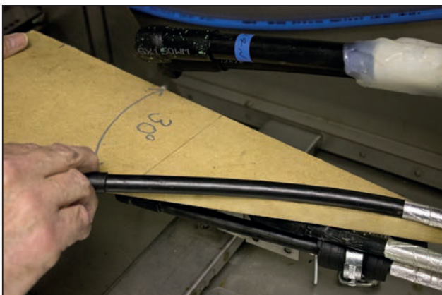
Image 3: Cable Bending
