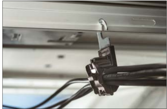
Ratchet P-Clamp Hanger applied to a solar panel.
